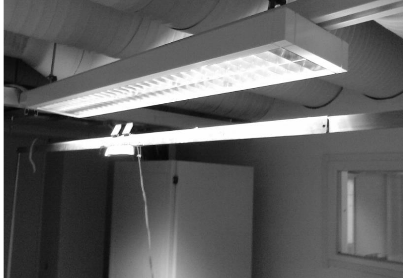
Figure 2.29 View of the final illumination configuration
