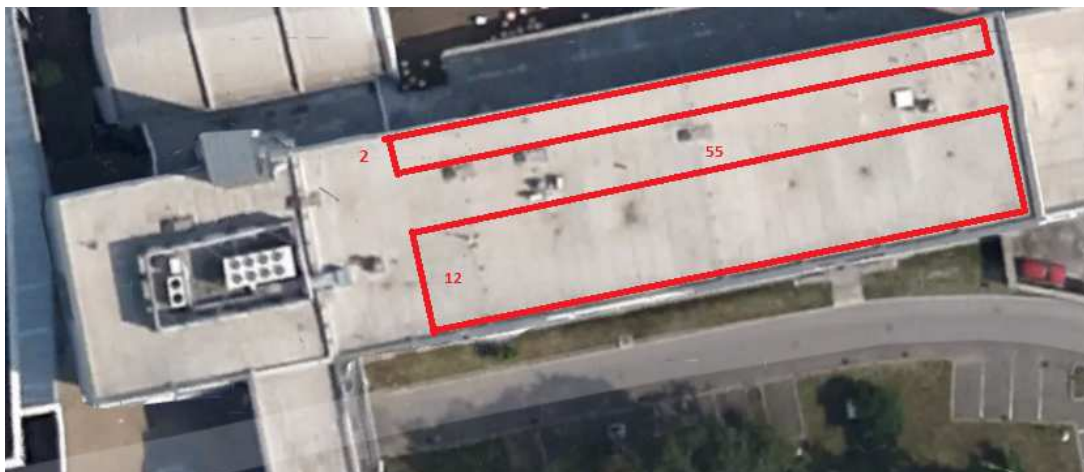
Figure 6. Top view of the zone 2 of the faculty building
