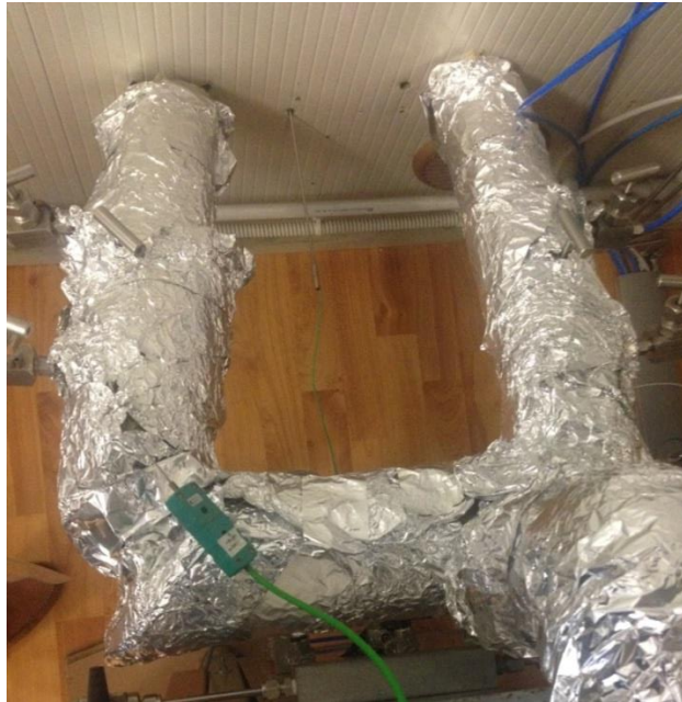
Figure 35: Test rig output pipes
