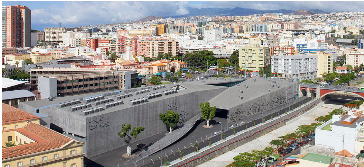
Img. 16: Vista general TEA.
