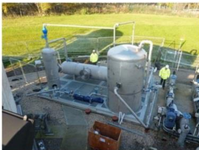
Figure 23. Full-scale plant of Cellruptor process.
