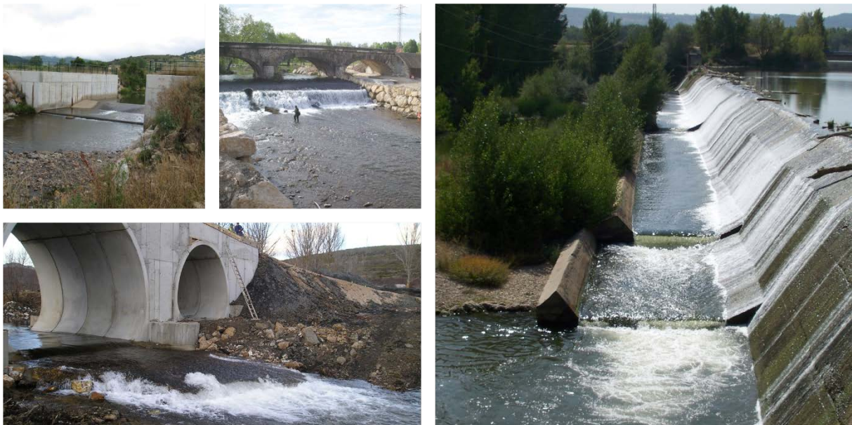
Figure 1. Cross sectional structures that may have a negative impact for fish migration: gauging stations, dams, weirs or bridges.
