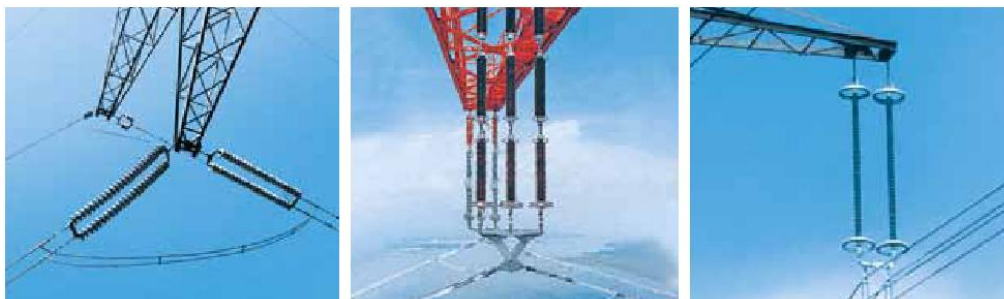
Example/Comparison of Insulator Application for a 400 kV Transmission Line
