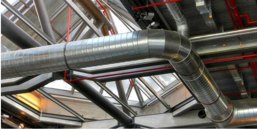
Figure 4.8. Circular ductwork
