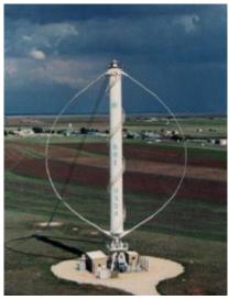
Figure 4.5.-Vertical axis turbine[6]
