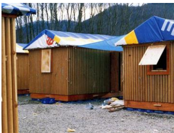
Paper log house, 1995. Shigeru Ban.
