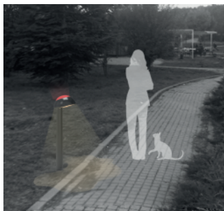
Bollard gives directional functional light to light up the road around Devrim area. Shape of the functional light is similar to acrylic layers on the pole top.
