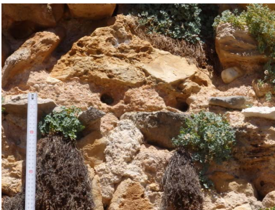
Fig. 5.6.71. Mechinal M3.10 de varillas pareadas [A.S.E. 23/7/2016]
