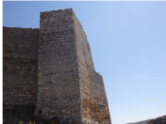
Fig. 5.3.63. Torre T11 [A.S.E. 8/7/2015].
