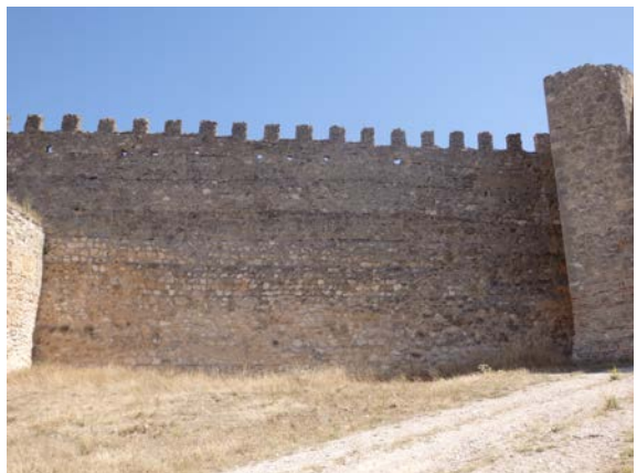
Fig. 5.3.53. Tramo T9-P3 [A.S.E. 8/7/2015].
