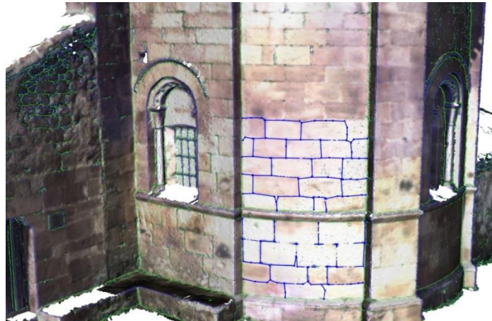
Fig. 5: Manual delineation outlining characteristics using the intrinsic color of the mesh corresponding to the church of Valberzoso (Palencia).
