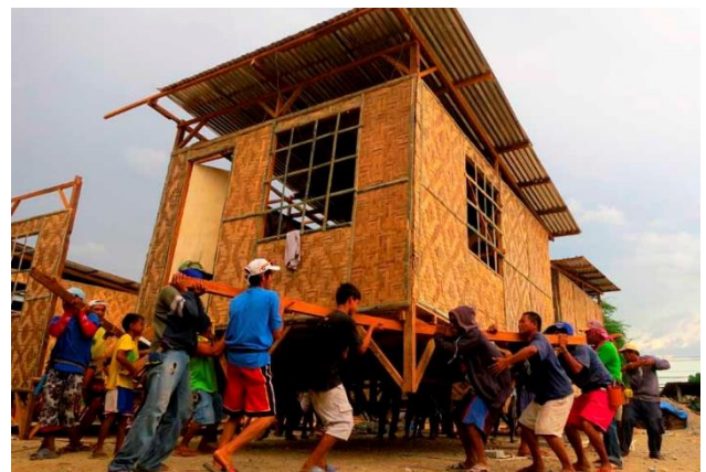
Photography 36. Transitional shelter for Philippines 2011 tropical storm. Model 02. Source: IFRCRCS, Post disaster shelter: Ten designs , Geneva, 2013. p 65.
