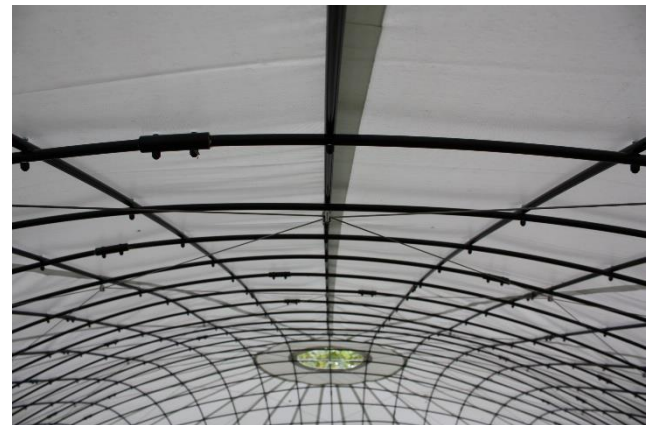
Photography 09. Sheltair emergency shelter. Inside view gridshell structure. Source: https://www.plataformaarquitectura.cl/cl/884525/membrana-reticular-economica-y-facil-de-usar-utiliza-cojines-rellenos-de-aire-para-la-construccion
