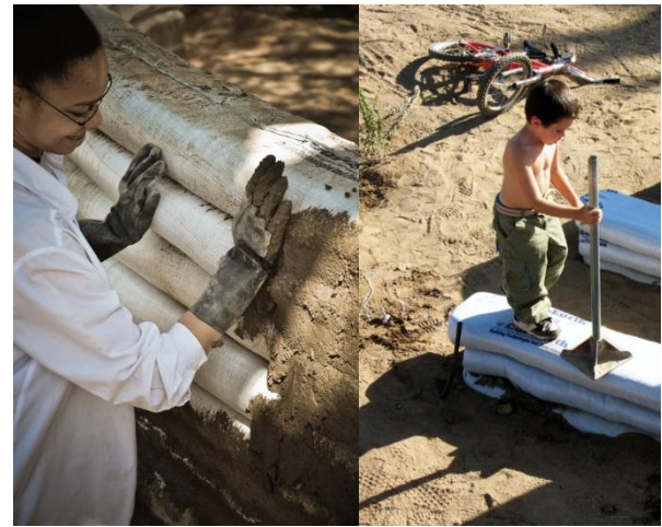
Photographies 48 and 49. Superadobe humanitarian project. Constructive process. Source: https://www.calearth.org/intro-superadobe
