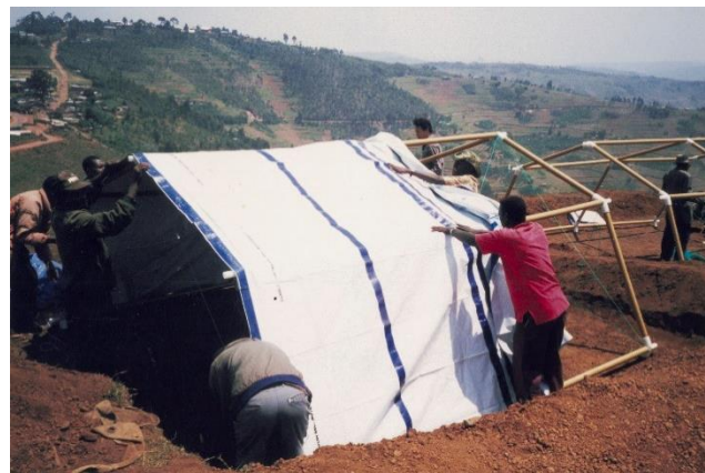
Photography 32. Paper emergency shelter. Covering the paper structure. Image© Shigeru Ban Architects.
