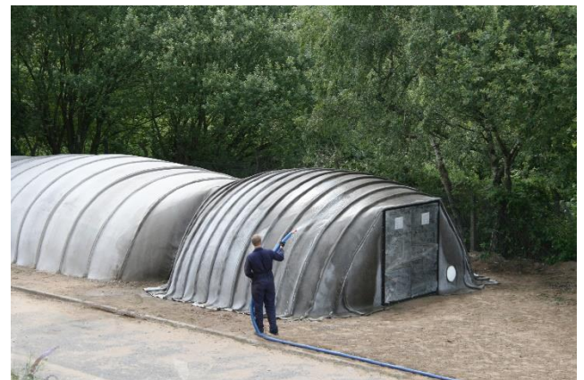
Photography 14. Concrete Canvas Shelter installation. Hydration process. Source: https://www.flickr.com/photos/_concretecanvas/sets/72157638403394195/
