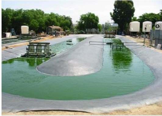
Figure 6. HRAP with a thick dividing section. In this picture, the water flows in a clockwise direction powered by two paddle wheels. (Credit: SARDI: South Australian Research and Development Institute)
