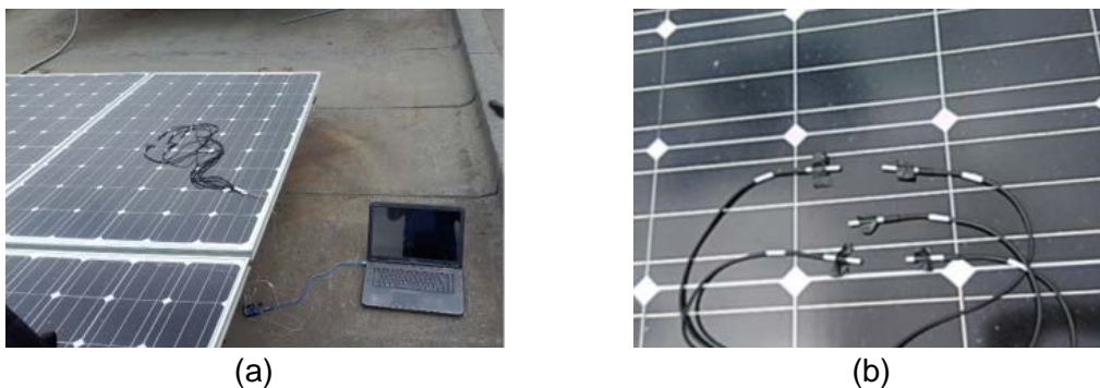
Figure 7: Temperature sensor matrix validation (a) Setup (b) Sensors deployed.
