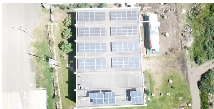
Figure 14: General view of the PV modules of the 35kWp at the University of Cuenca.
