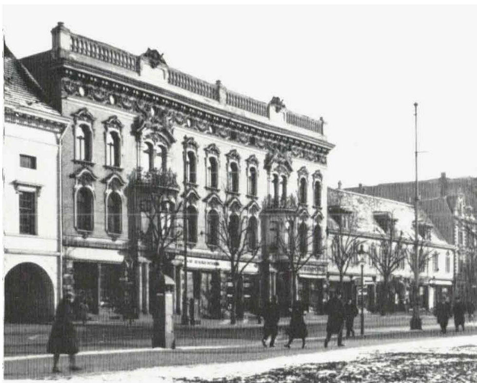
109, 110. Under Mies, Eduard Ludwig redesigned an existing department store in Dessau, Germany, 1932. The store and its proposed new facade.
