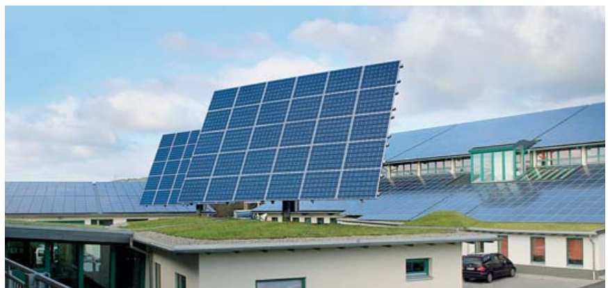
sonnen_system trackers on the roof of Kirchner Solar Group headquarters
