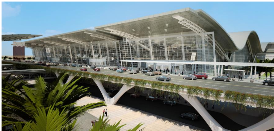
Fig.17: Proyecto del Hamad International Airport Passenger Terminal Comple, realizado con plataforma BIM Fuente: http://www.hok.com/design/type/aviation-transportation/hamad-international-airport/
