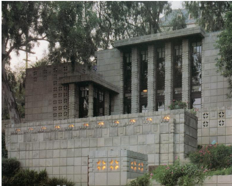
Frank Lloyd Wright, Storer House , Hollywood, 1923. 81
