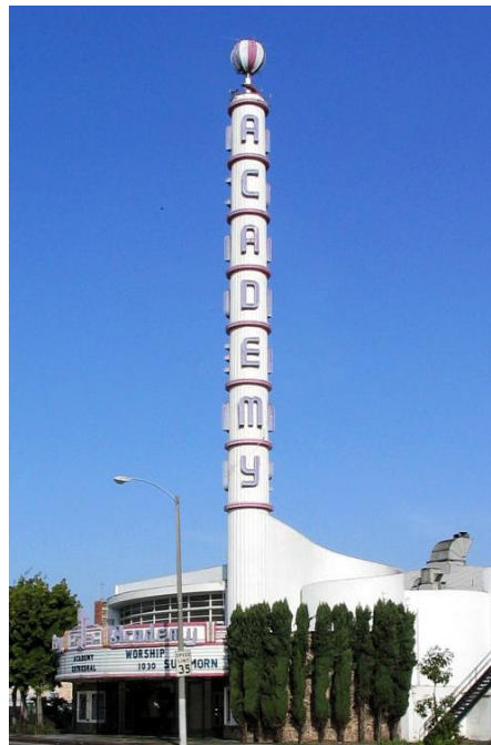
Charles Lee, Academy Theatre , Inglewood, Los Angeles, 1938. 242
