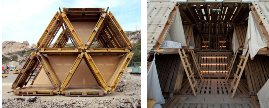
Figuras 85 y 86. Hexa Structure. Refugio modular. Fuente: J.SANCHEZ, P. SÁNCHEZ, J. ARIAS. Palet Project: Building with palets.
