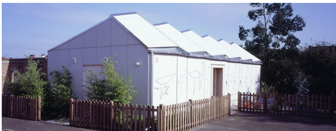
Ilustración 24. Westborough Primary School. Fuente. http://www.burohappold.com/projects/project/west-borough-primary-school-cardboard-building-73/
