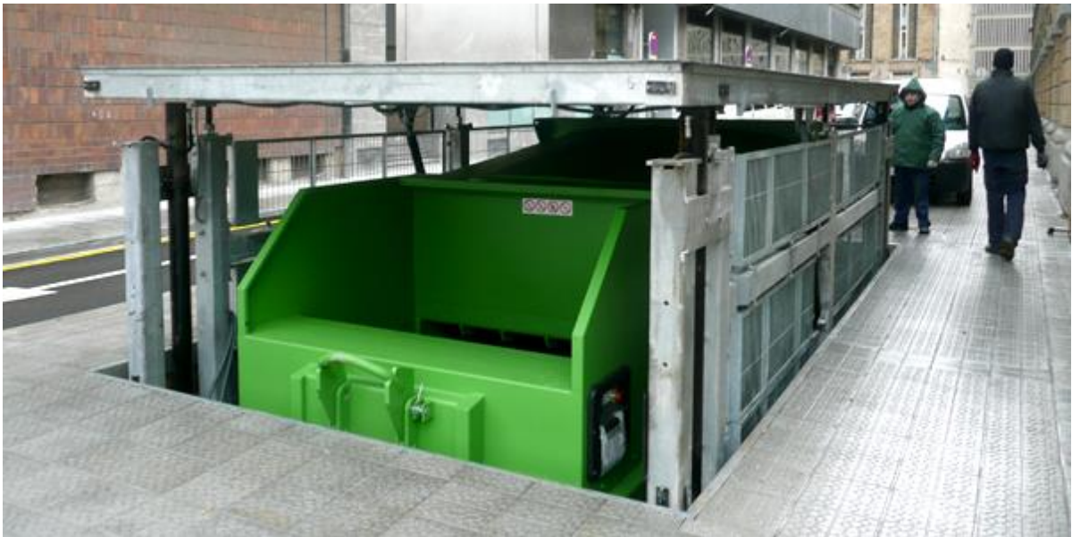
Pic 6. Underground Compactor
