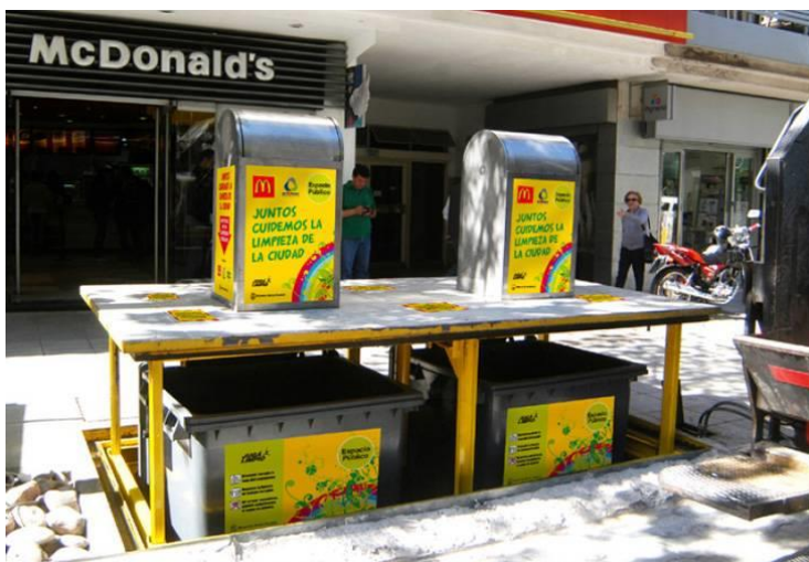
Pic 9. Underground rise containers
