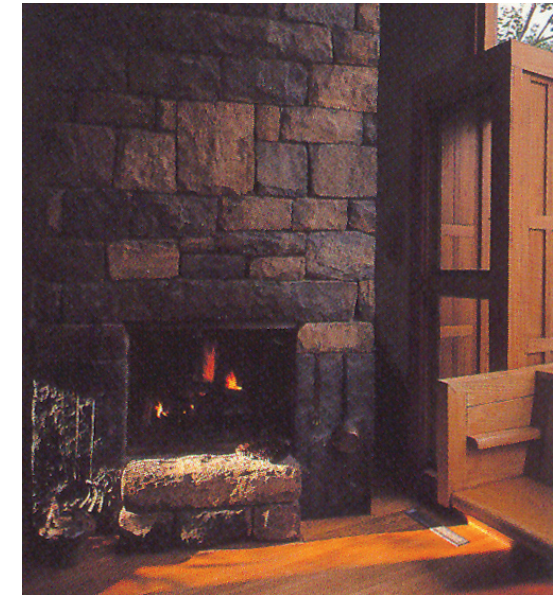
3.648. Louis Kahn, chimenea de la casa Fisher.
