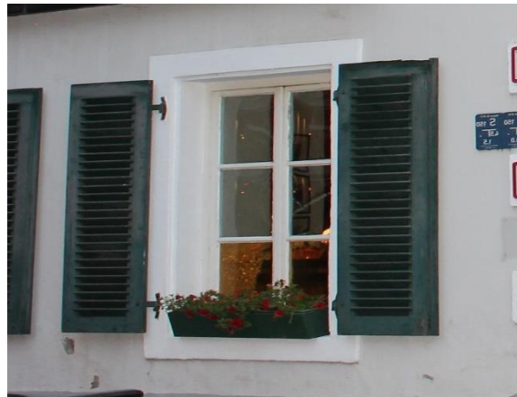
Window shutter tipe 1 photo
