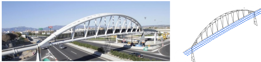
Fig. 1: Footbridge under study: photograph and numerical FE model
