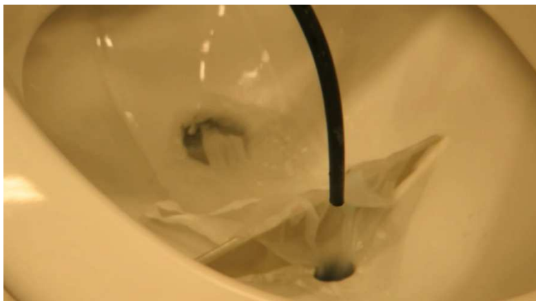
Figure 28 Toilet paper problem in EVAC toilet
