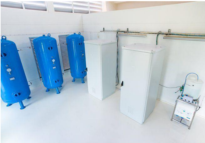
Fig 2. Example of a hydrogen-based microgrid ( https://www.curbed.com/2016/1/22/10844376/solar-powered-hydrogen-home-thailand )
