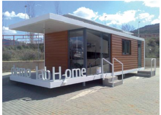
Fig 3. Smart house powered by renewable energies and a hydrogen-based microgrid in the CNH2, Spain
