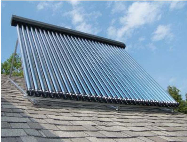
PICTURE 17. Installed heat-pipe collector. (sunpower-solar.com)
