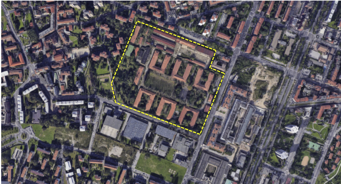
Fig. 1. View of the Mameli barracks.
