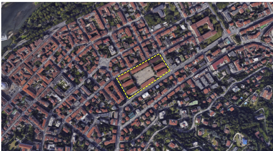
Fig. 5. View of the Alessandro La Marmora barracks. Source: delimitation of the area starting from Google Maps, 2018.
