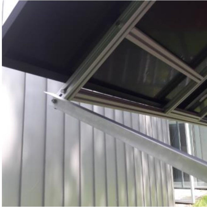
Figure 43. Lock beams for the Lateral Frame in The Moving Lab.
