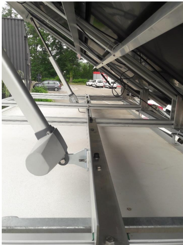
Figure 36. Actuator fulcrum in The Moving Lab.
