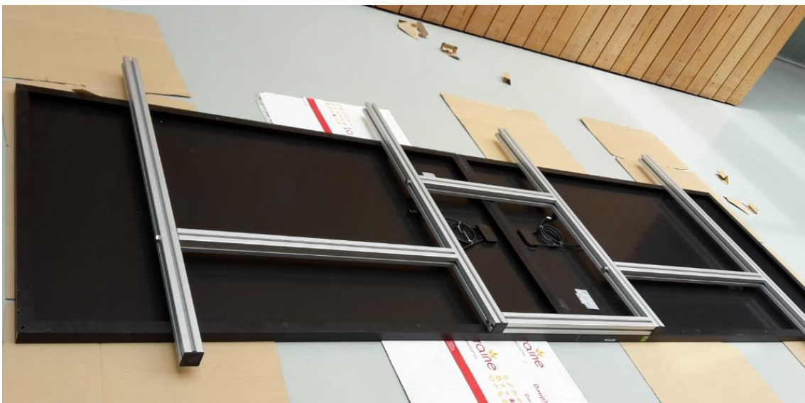
Figure 53. Construction of the Lateral Panels detail.
