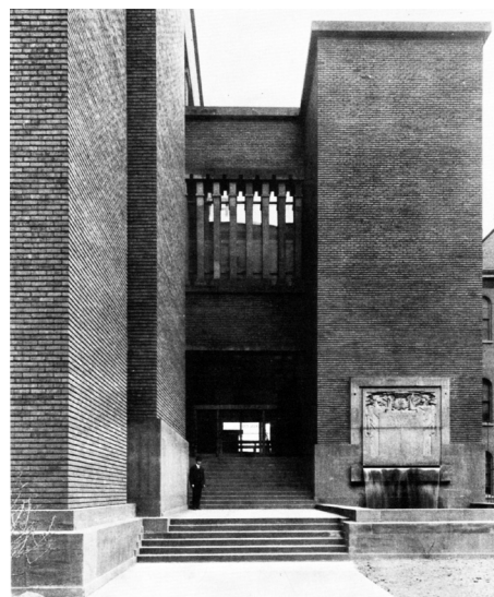
5 Anexo, entrada por Seneca Street. [Jack Quinan. Frank Lloyd Wright's Larkin Building. Myth and Fact ]
