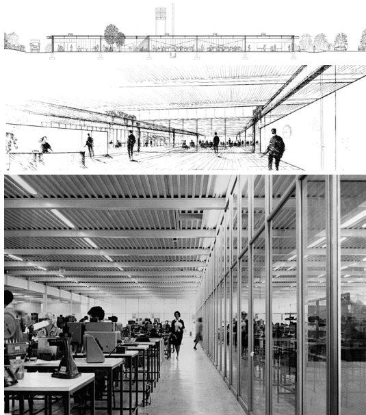
Reliance Controls Electronics Factory, Swindon, 1965/66.
