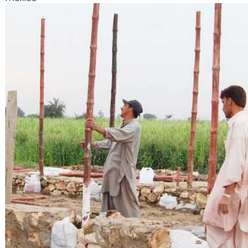
Figura 06: Imagen de la construcción del orfanato ABC, OAC. Fuente: https://www.dezeen.com/2016/03/10/architecture-for-humanity-relaunches-as-open-architecture-collaborative-humanitarian-charity/
