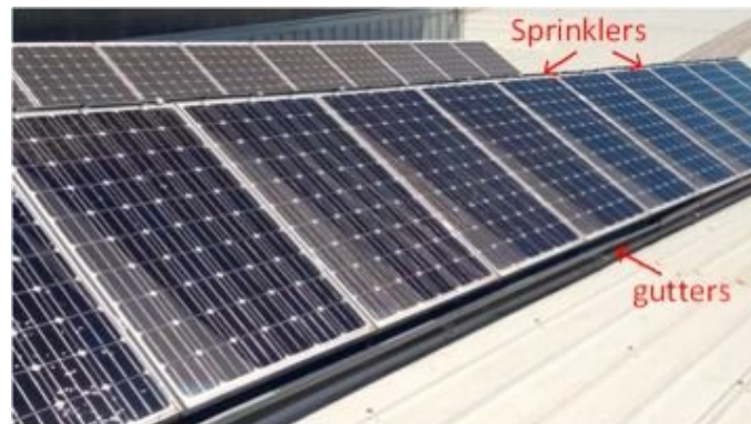
Figure 23. Visual layout of water sprinkler cooling system (Castanheira A., Fernandes J., Branco C., 2018)
