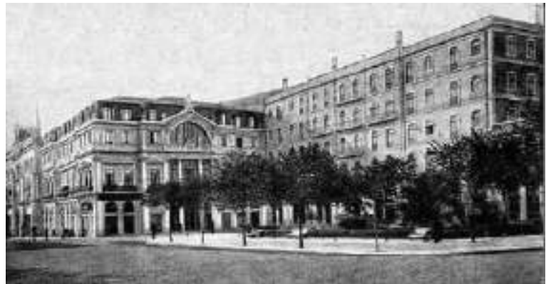
Fig. 13 Hotel Avenida Palace
