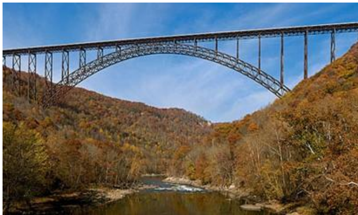
Figura 38: Puente George. Virginia.
