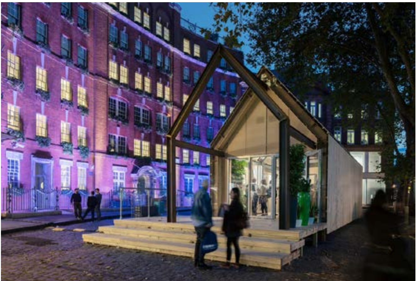
Imagen 37: The Circular Building . Arup Associates. Fuente: ArchDaily, página web: https://www.archdaily.com/868121/arup-designs-prototype-building-based-on-circular-economy-principles
