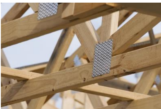
Figura 17. Unión mediante placa clavo. https://www.newhomereview.com.au/glossary/gusset-plate/
