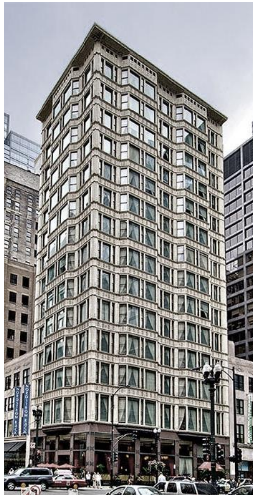
Figura 54. Fachada Reliance Building
