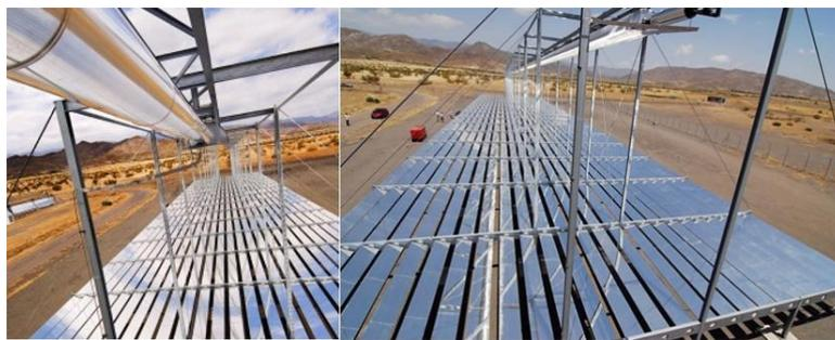
Figure 18: Linear Fresnel MAN collector from Almería Solar Platform (PSA) [36].
