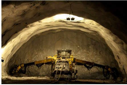
(a) Jumbo and excavation front
