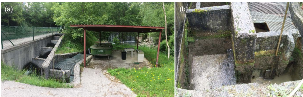
Figure 12. Marín River: (a) fishway, measure station (waiting tank and measure table) and the weir at the background of the picture; (b) detail of a portable gate (empty fishway). Source: GEA-Ecohidráulica.
