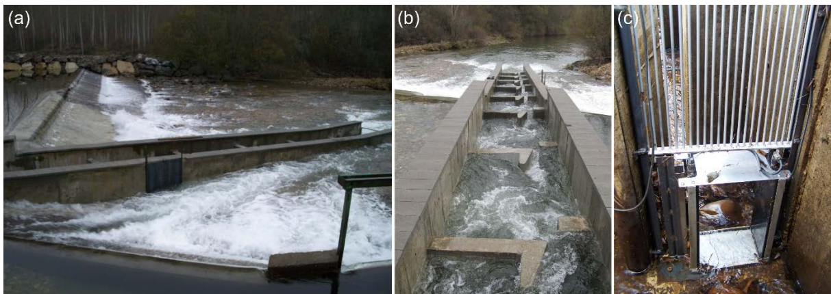
Figure 10. Porma River: (a) dam and fishway; (b) inside of the fishway; (c) fish counter (VAKI Riverwatcher) installed in the most upstream slot of the fishway. Source: GEA-Ecohidráulica.
