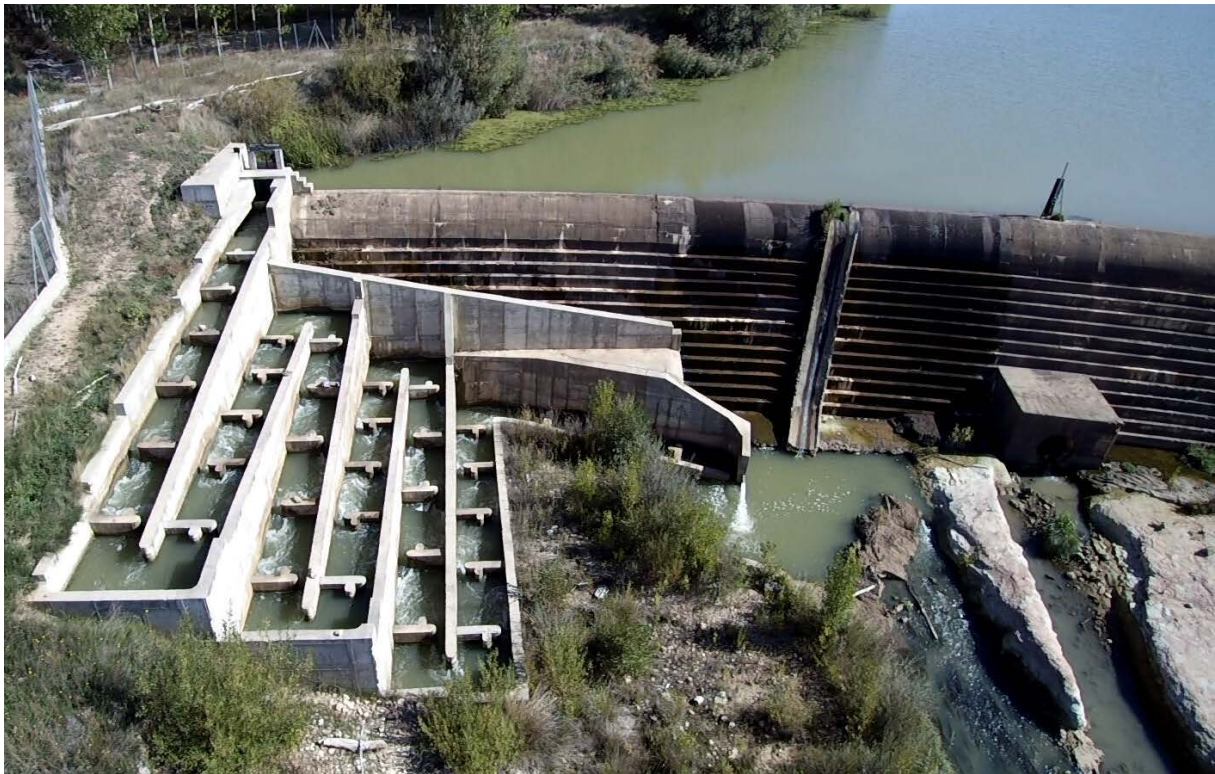
Figure 6. Stepped fishway (submerged notch and orifice type) in Guma dam (Duero River, Spain). Source: GEA-Ecohidráulica.
