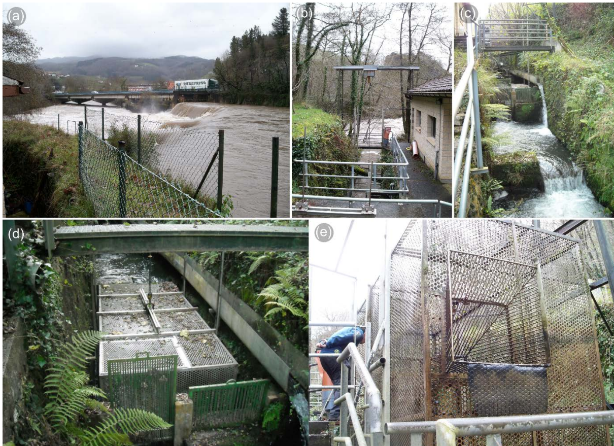
Figure 13. Bidasoa River: (a) weir; (b) monitoring station (stepped fishway and fish lift); (c) stepped fishway; (d) cage of the fish lift inside the upper pool of the stepped fishway; (e) detail of funnel to enter into the cage of the fish lift. Source: GEA-Ecohidráulica.
