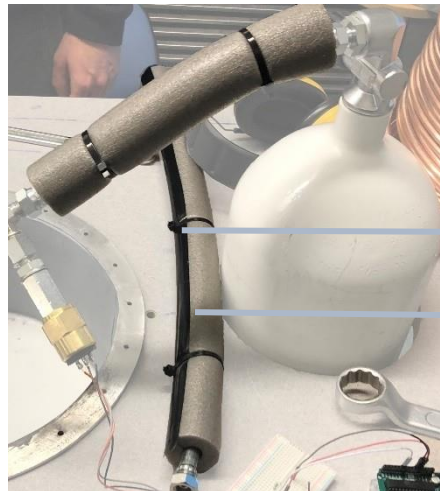
Figure 74 Construction of insulation
