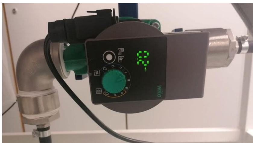
Figure 36 Final assembly of the pump
