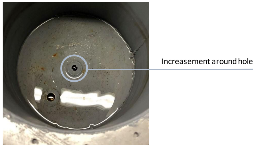
Figure 20 Still water in casing of TES
