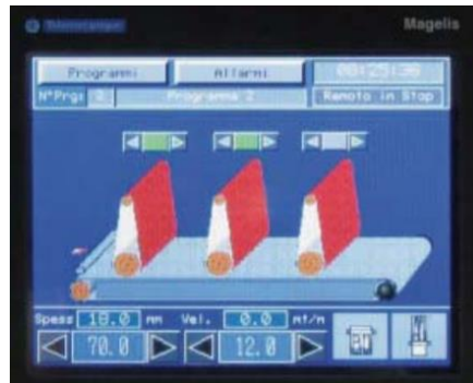
Figure 11.6. Example of what can be seen in the screen of the PLC in the Costa Levigatrici Series 6 calibrating sanding machines.
