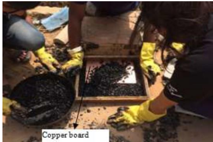
Figure 19. Copper board embedded in pavement [26]
