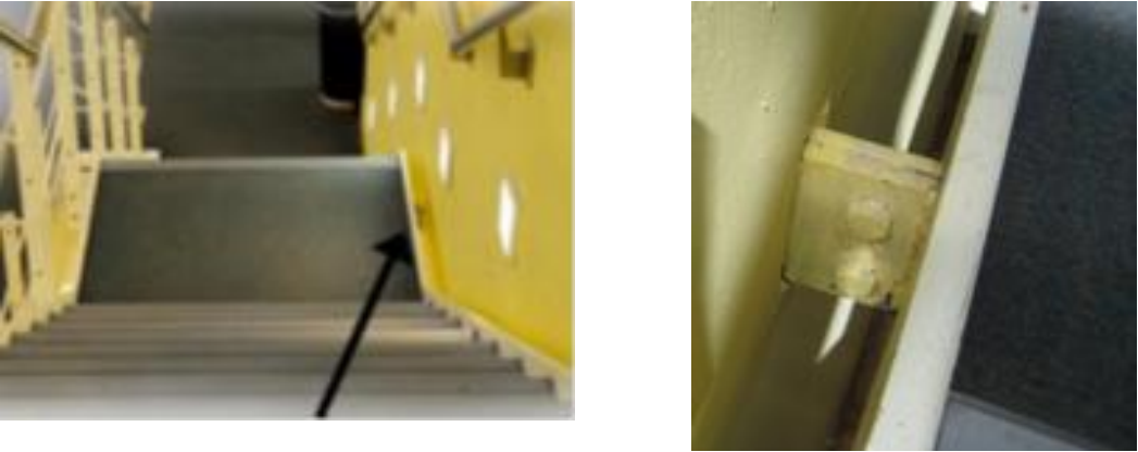
side support of the staircase
