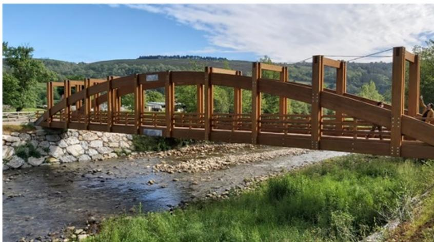
**Figure 1.** Pedestrian walkway built using laminated wood in the town of Cieza (Cantabria).
