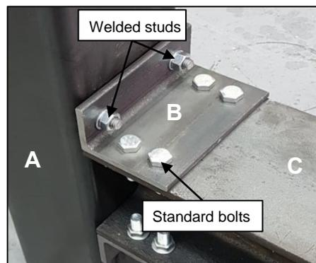
**Figure 1.** Example of the beam-to column joint assembled with threaded welded studs. A: hollow-section column. B: angle cleat. C: open-section beam.
