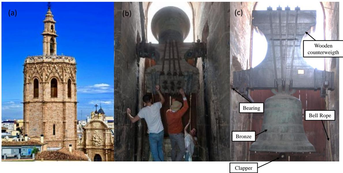
**Figure 1.** (a)- El Micalet bell tower. (b)- Bell ringers ringing the bell manually (c)- El Jaume bell before the collapse.
