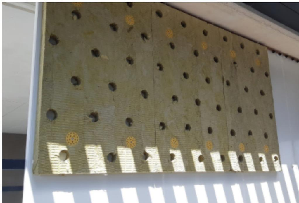
Figura 3. Panel de lana de roca (Fuente: [www.singulargreen.com](http://www.singulargreen.com))
