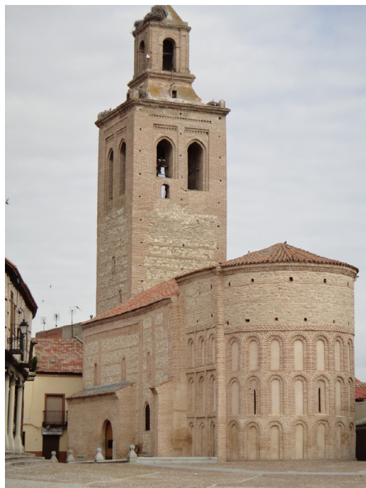
Fig. 2. Church of Santa María la Mayor in Arévalo, Ávila, Spain.
